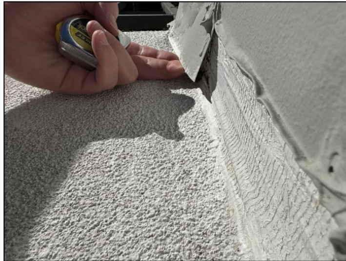
lifted flashing
