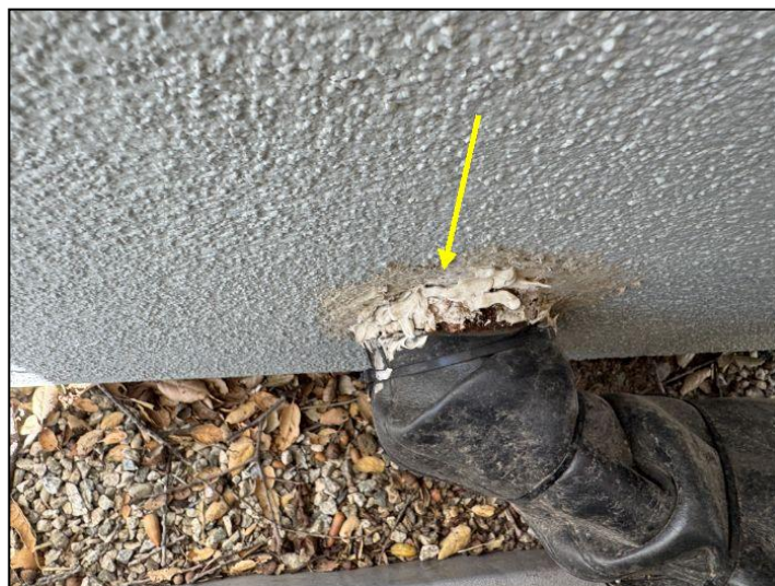
substandard seal
