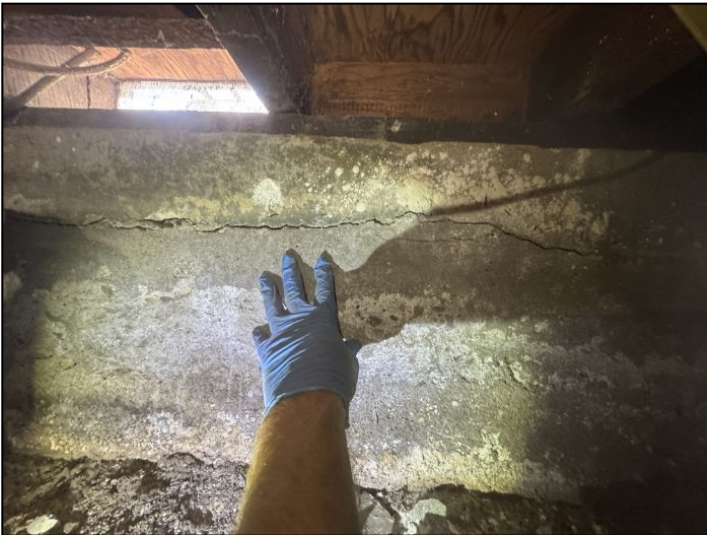
horizontal crack
