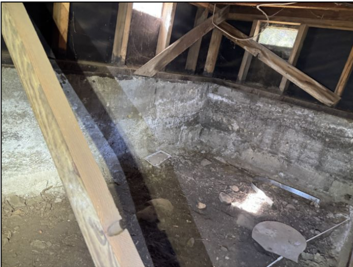
efflorescence
