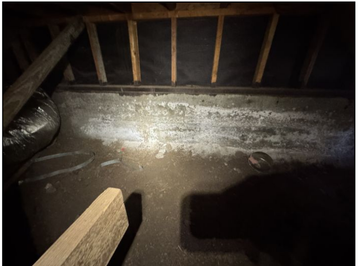
efflorescence
