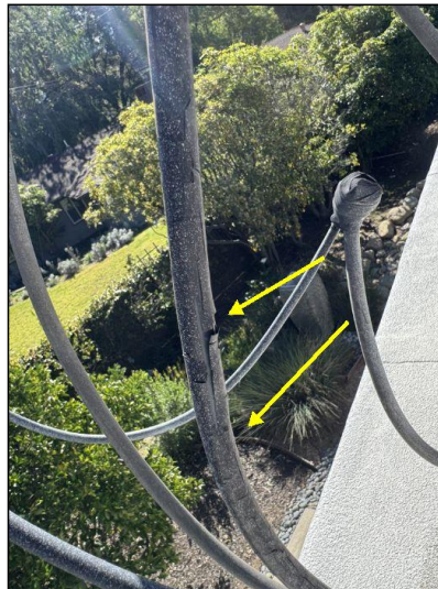
damaged conductors
