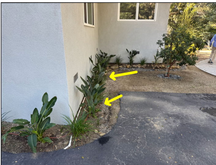
Poor grading
