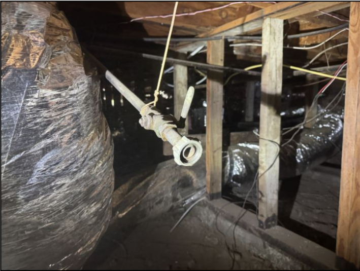
leaking plumbing in crawlspace
