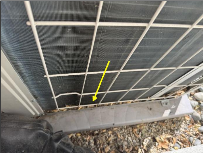
clean debris from unit
