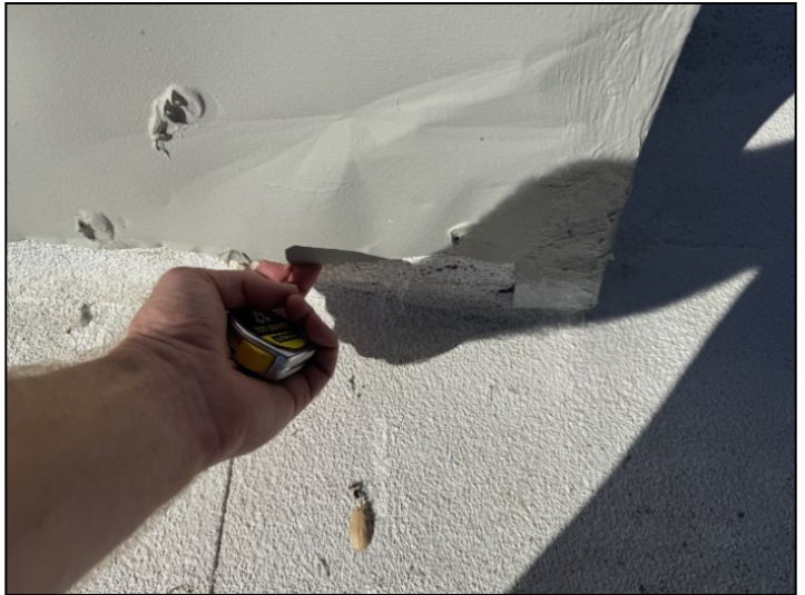
lifted flashing
