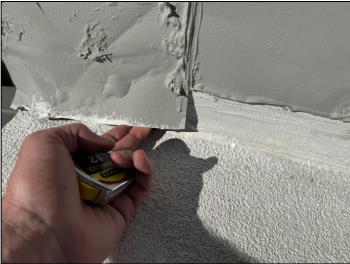
lifted flashing
