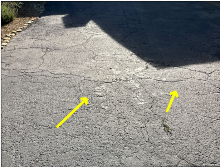
Moderate cracks
