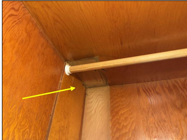
patching of closet ceiling
