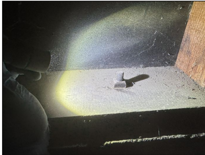
original foundation bolts
