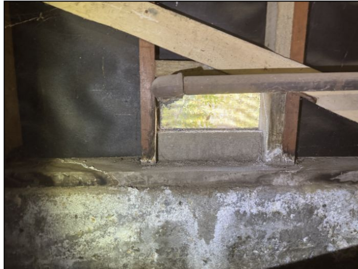
horizontal crack
