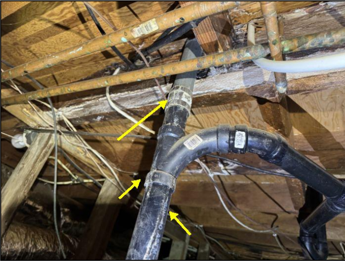
leaking plumbing in crawlspace
