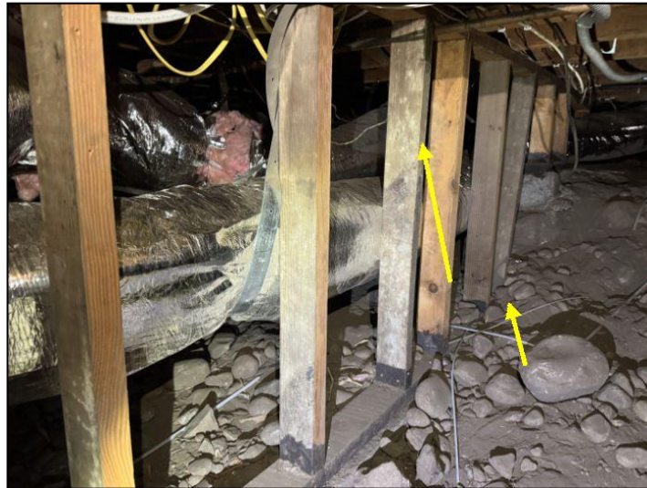
possible growth/soil contact
