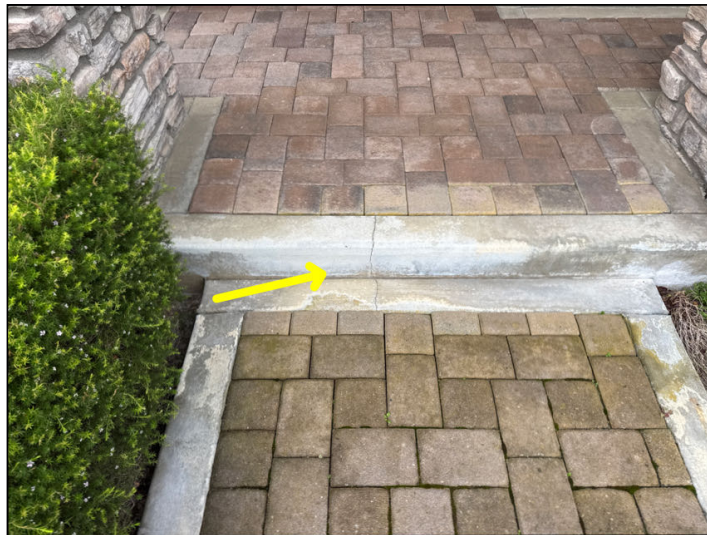
minor cracking
