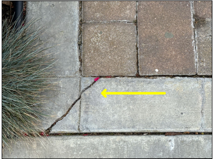
minor cracking
