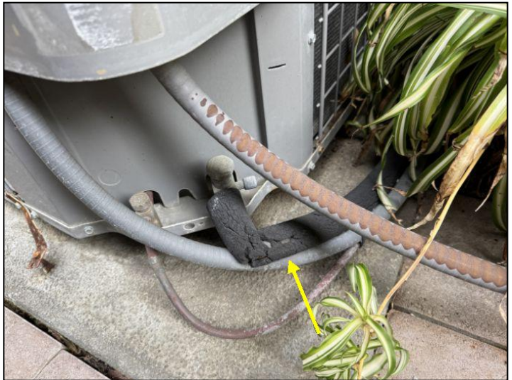
insulation damage
