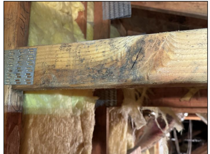
staining/possible microbial growth
