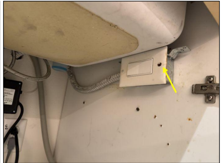
unknown function- missing screw
