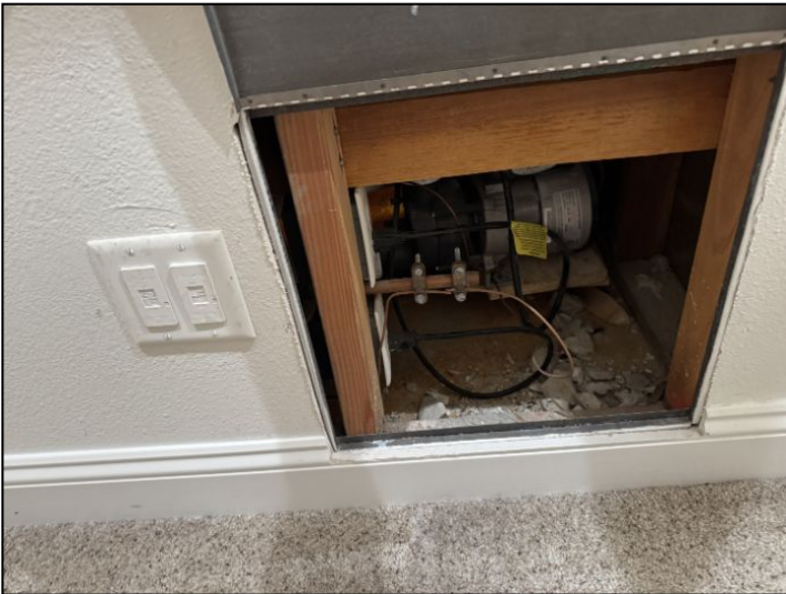
GFCI for tub
