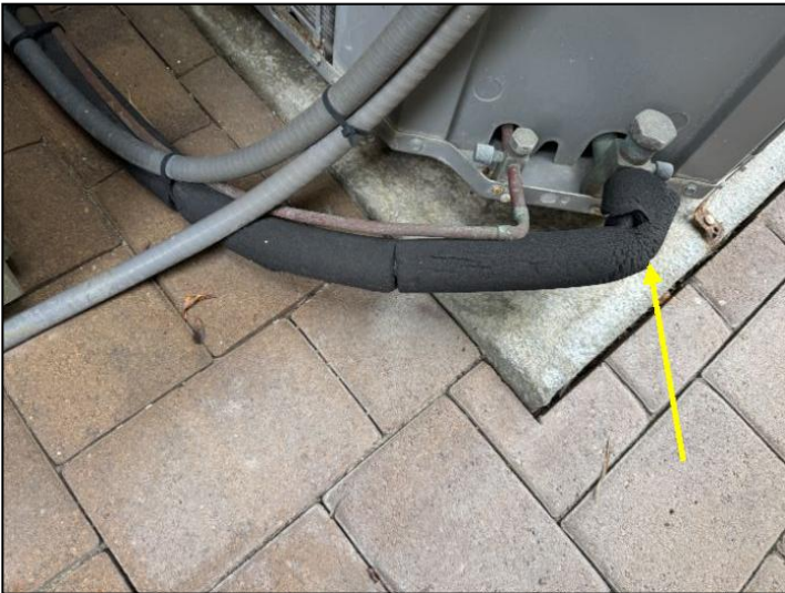
damaged insulation
