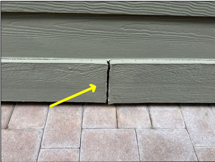
Seal gap - cover for unknown.
