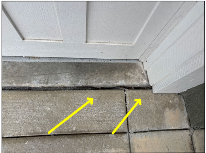
failing seal
