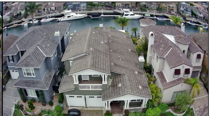
overall photo for client
