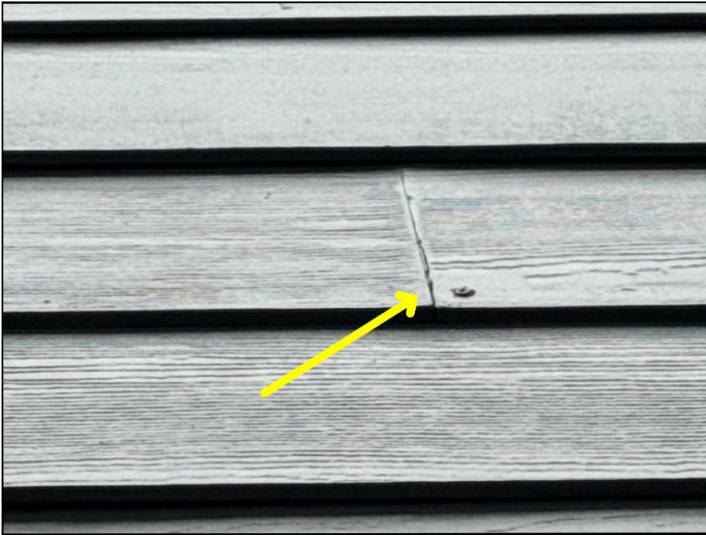
Seal gap - cover for unknown.
