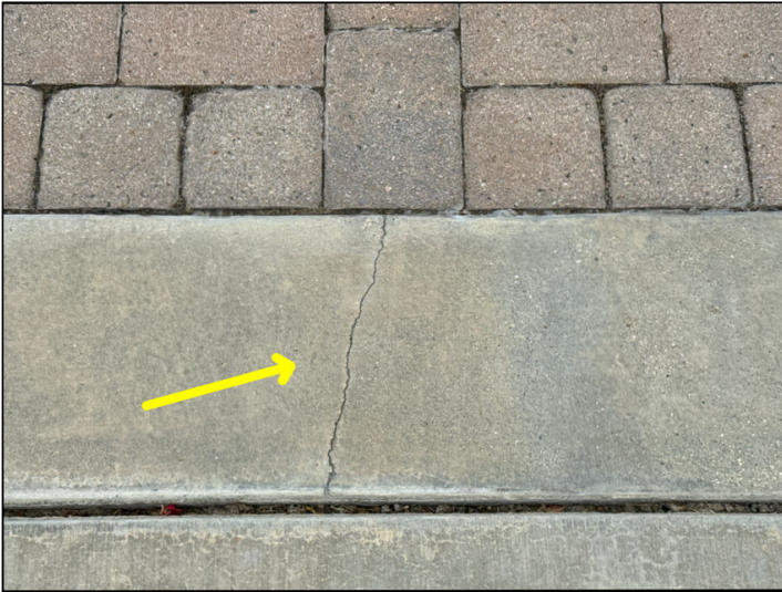
Minor cracking
