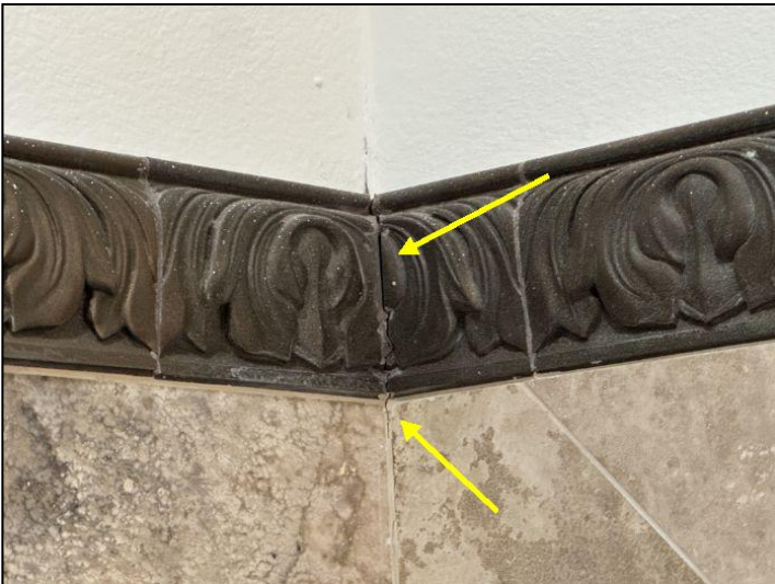
seal cracks
