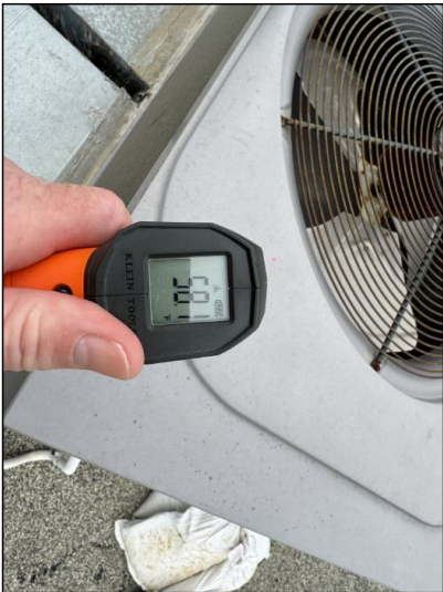
58 degrees did not run cooling cycle
