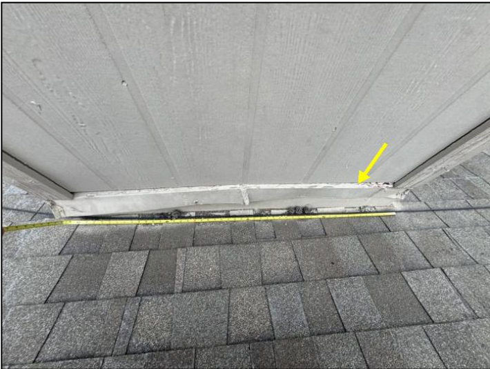
damage to flashing behind chimney-cricket recommended
