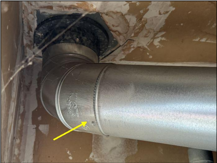
missing fasteners
