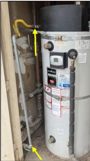
no sediment trap/use of white teflon tape
