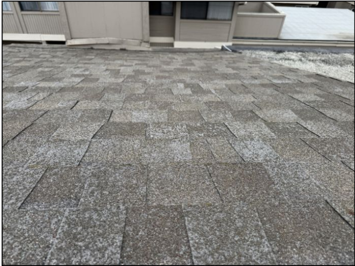
exposed fiberglass
