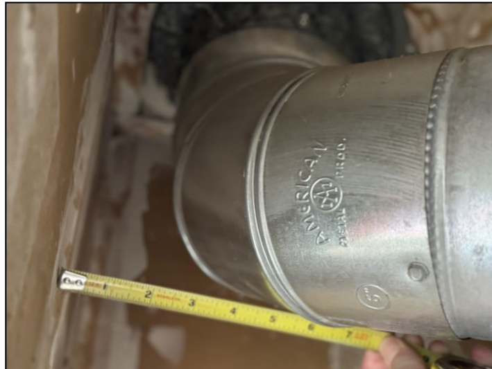
clearance to combustibles single walled flue
