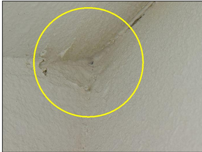
inside closet near garage
