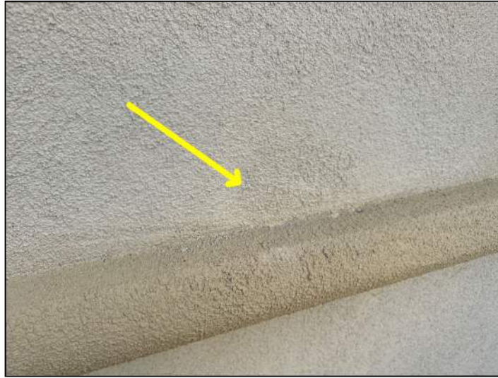
exterior patch job
