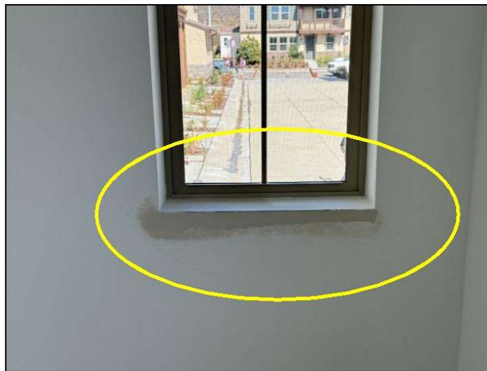
patch in progress
