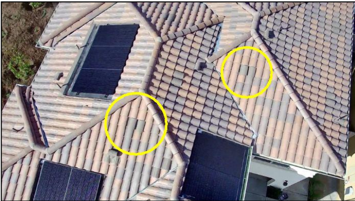
slightly out of place tiles
